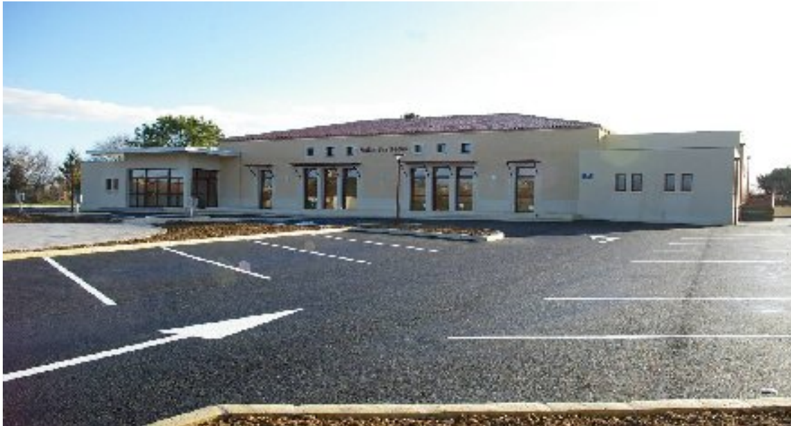
Un parking de 50 emplacements.
